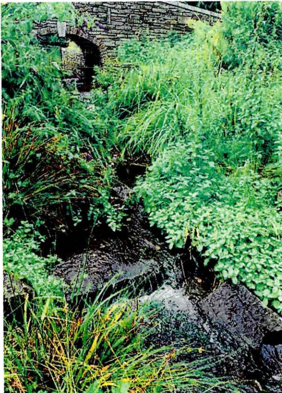
5. Photo of the watercourse exiting the pond on the other side of the stone bridge:
